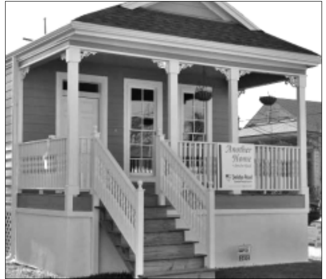
A completed Jericho Road house in New Orleans. Come be a part of this amazing Katrina recovery ministry.
