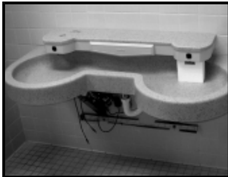
New tile and automatic sinks being installed
